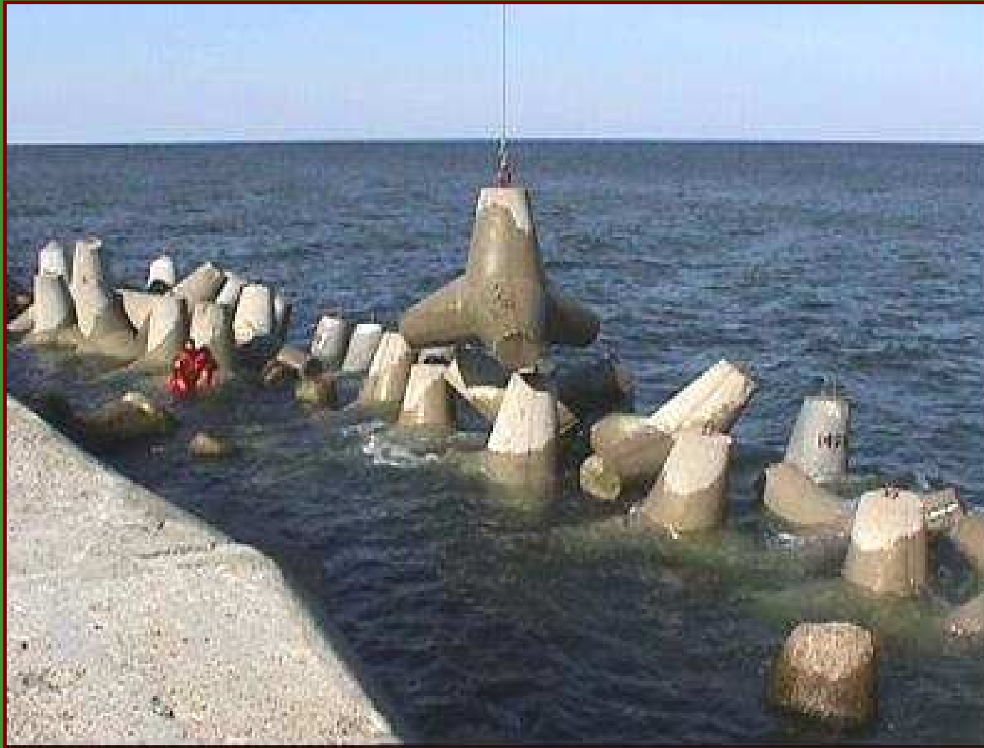
Reconstruction of armour at Wladyslawowo harbour breakwater in September 2003
