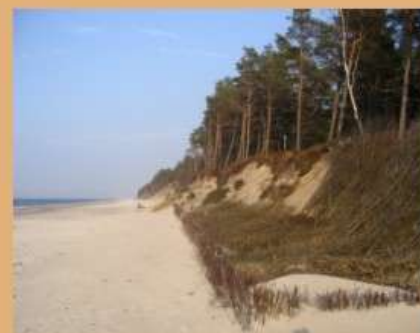
Fascine dune-forming fences and dune facing made by services of the Maritime Office in Gdynia
