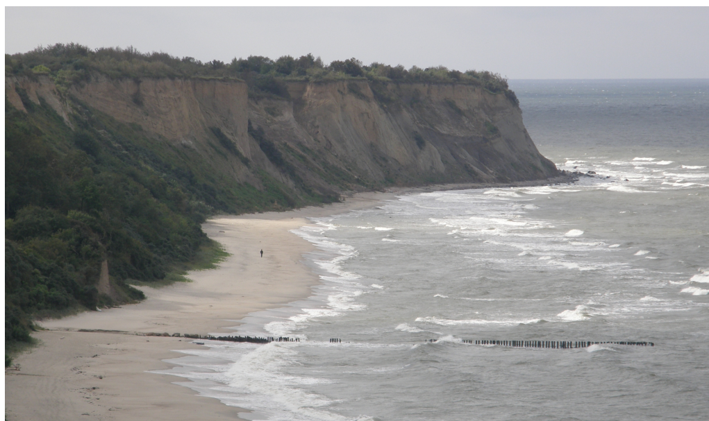
Fig. 6. The single groin near Donskoye (northern part of the western coast of the Sambia Peninsula) constructed in 1938 for protection of the wastewater pipeline outlet
