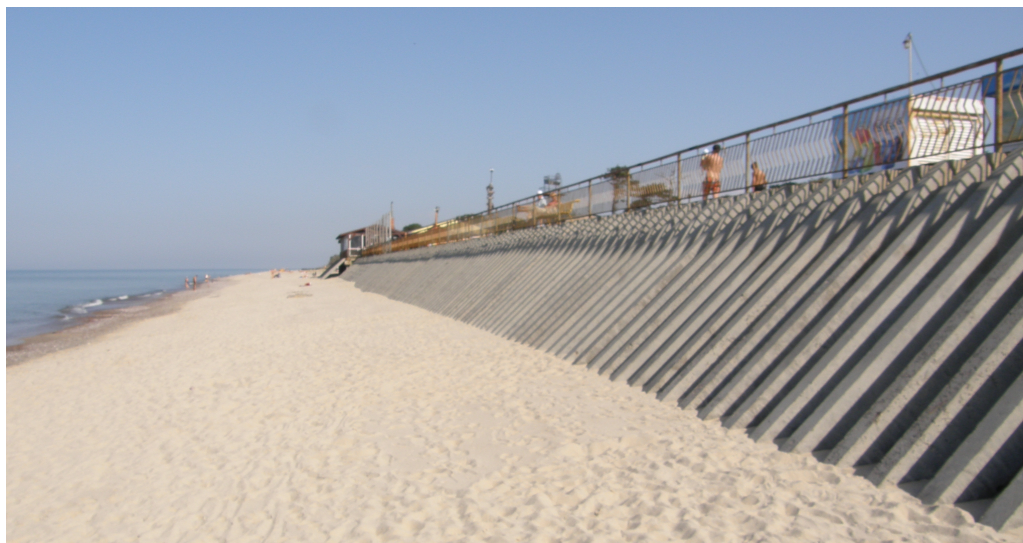
Fig. 11. A massive permeable revetment with pavement on top in Lesnoy, built in 1995
