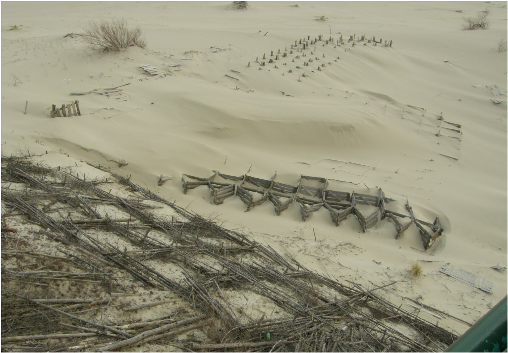
Fig. 12. Stabilisation of quicksand on the Curonian Spit
