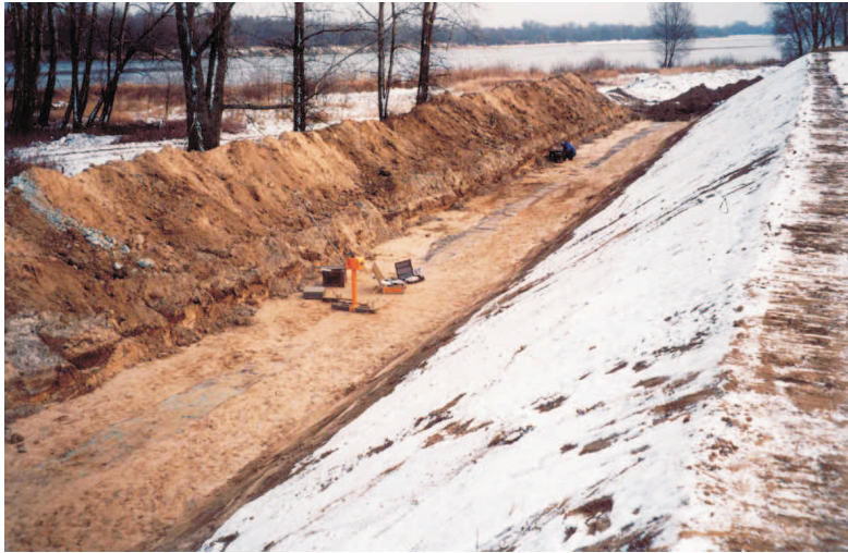
Fig. 4. View of the experimental section
